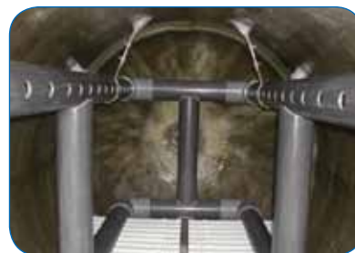
Looped lateral system - Inside view
